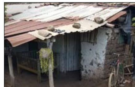
A roof of discarded sheet metal and rocks gives little protection during Honduran storms.
